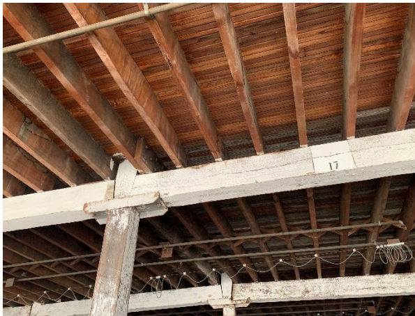
Figure 23: Existing timber floors within Woolstore 1 are to be retained in situ, with the underside of the floor visible from the level below the floor. (Source: CN, 6/10/2020)
